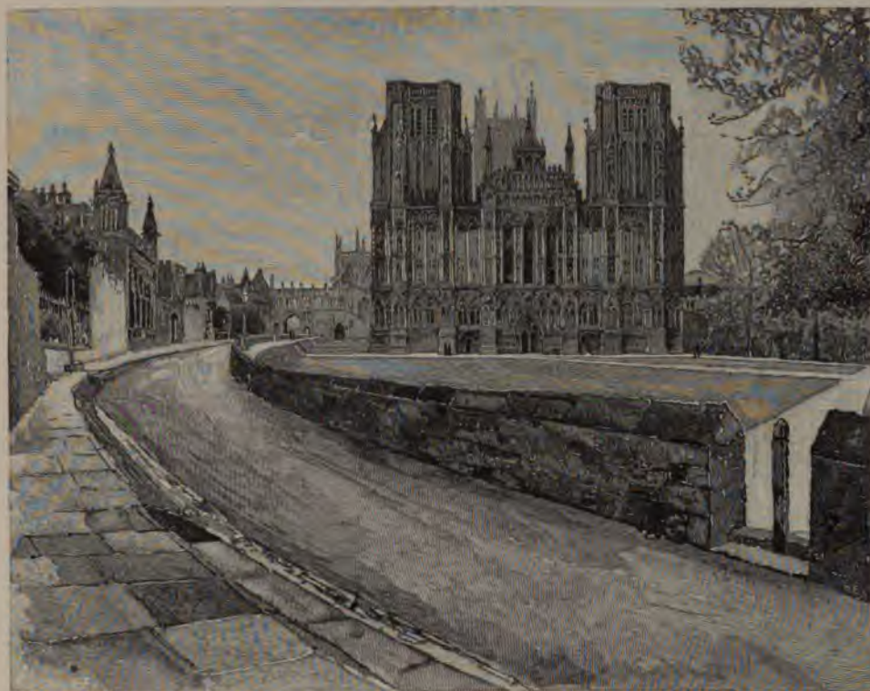
THE WEST FRONT OF THE CATHEDRAL.
